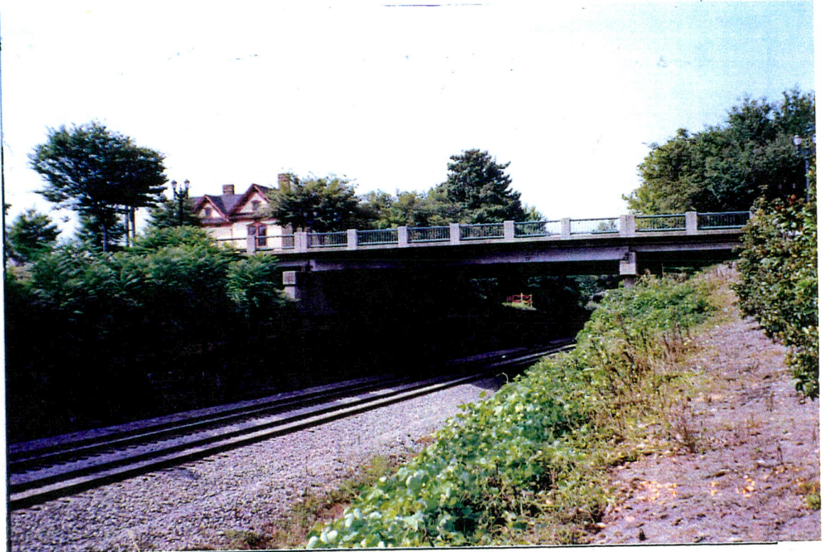
Bridge No. 381 View from east to west
