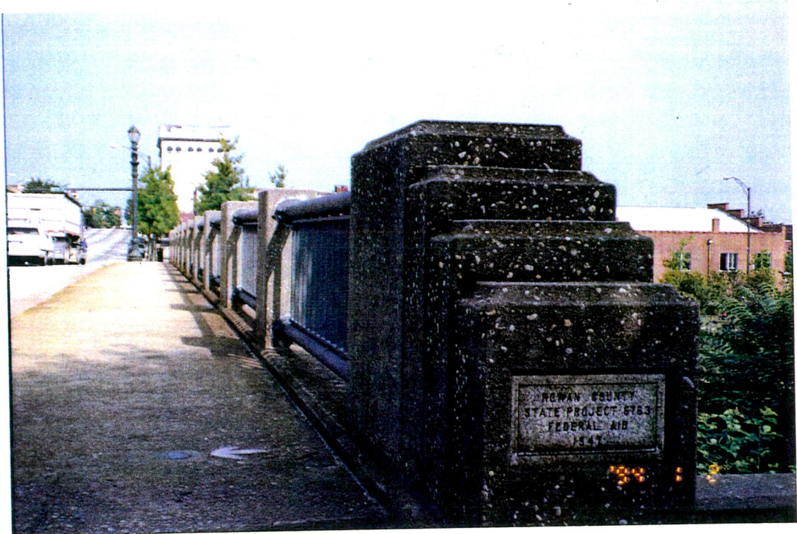
Bridge No. 381 Stacked pier and plaque View looking north
