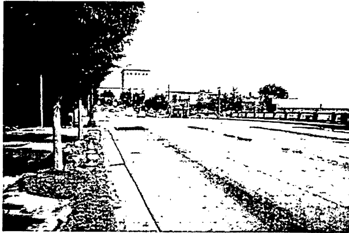
Fig. 21 – East Innes Street, looking West from the Innes Street Bridge
