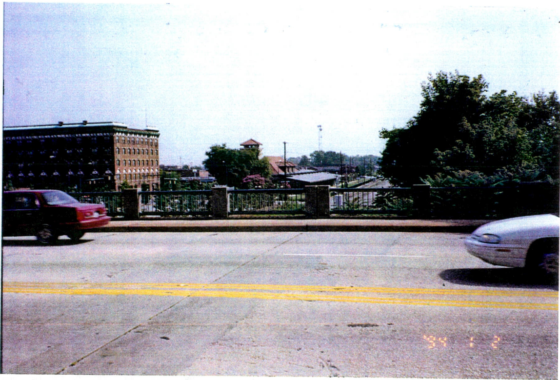
Bridge No. 381 View from west side of bridge Depot and former Yadkin Hotel in the distance
