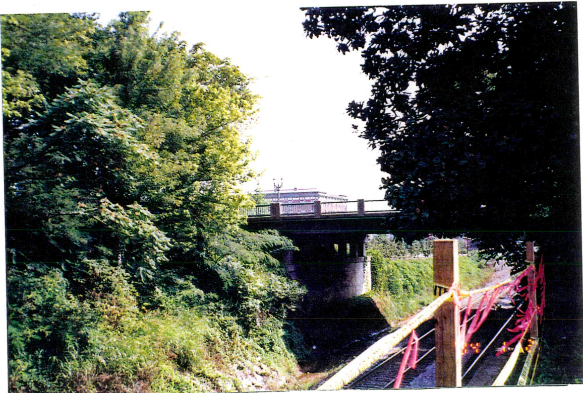
Bridge No. 381 View west to east
