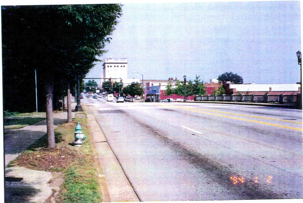
Bridge No. 381 View from Bernhardt House looking north
